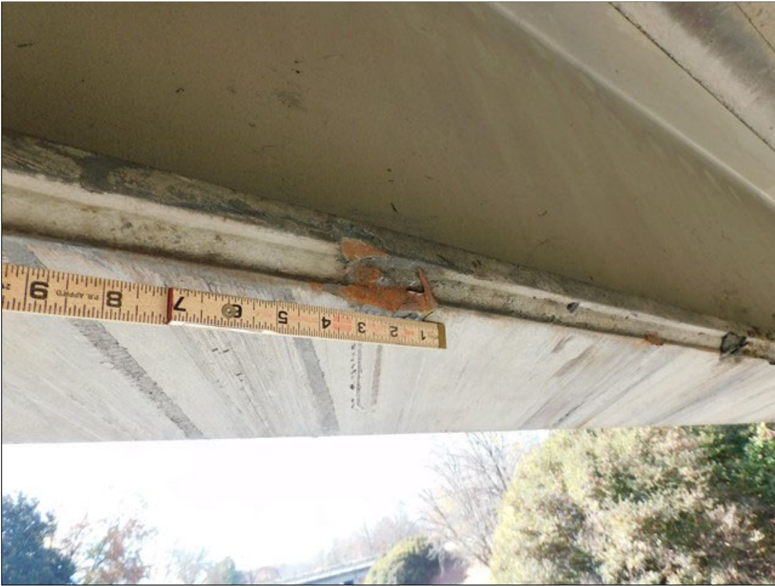
Span 2 Beam 10: IMPACT-11/19/2025- PRIOR DAMAGE; LOCATED 21.2 FEET FROM INTERIOR BENT 1 - AREA 8 FEET LONG DEFLECTED TOWARDS SOUTH 1.25 INCHES WITH SEGMENT OF BOTTOM FLANGE DEFLECTED UPWARDS 1.5 INCHES - ALONG BOTTOM FLANGE AT MID SPAN, AREA OF IMPACT DAMAGE [8 FOOT LONG] WITH AREA OF DELECTION [1/4 INCH X 3 FOOT LONG] ON SOUTH FACE AND DEFLECTED UP [1.25 INCH X 4 FOOT LONG] ON NORTH FACE.
