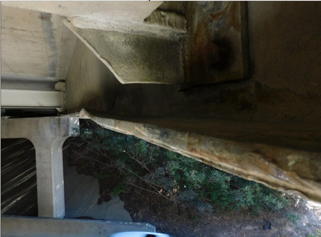
Span 2 Beam 10: IMPACT-11/19/2025- PRIOR DAMAGE; LOCATED 21.2 FEET FROM INTERIOR BENT 1 - AREA 8 FEET LONG DEFLECTED TOWARDS SOUTH 1.25 INCHES WITH SEGMENT OF BOTTOM FLANGE DEFLECTED UPWARDS 1.5 INCHES - ALONG BOTTOM FLANGE AT MID SPAN, AREA OF IMPACT DAMAGE [8 FOOT LONG] WITH AREA OF DELECTION [1/4 INCH X 3 FOOT LONG] ON SOUTH FACE AND DEFLECTED UP [1.25 INCH X 4 FOOT LONG] ON NORTH FACE.
